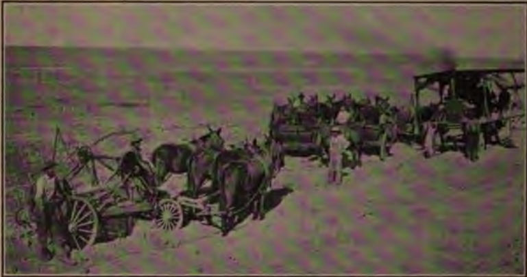
A Series of Maney Scrapers with Traction Engine Auxiliary for Loading. Figure 9.
